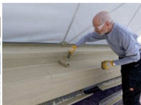
KEMPEROL® Waterproofing only came into contact with the special plastic fabric at the junction points, which were waterproofed separately. Application: The first layer of KEMPEROL® is applied, a reinforcing fleece is then embedded within this base coat, a second layer of KEMPEROL® is immediately applied as the top coat to fully saturate the wet fleece.
