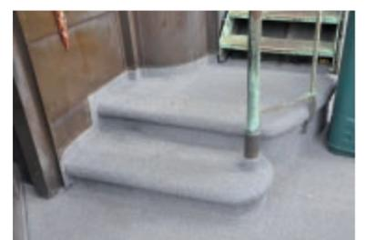
The observation deck of the Hamburg Michel was effectively waterproofed using KEMPEROL® and given hard-wearing-coating using KEMPERDUR®. Round shapes and many complex details-ideal for the application of liquid applied waterproofing
