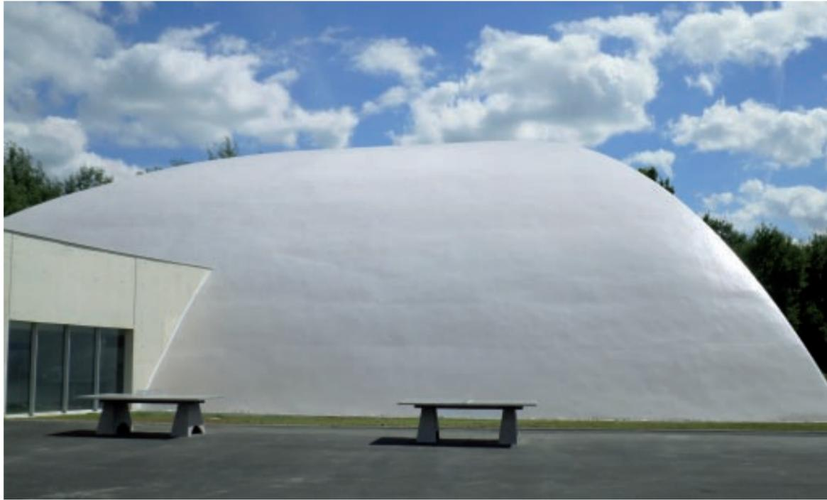
For purely visual effects the KEMPEROL® surface is covered with a colour-stable white KEMPERDUR® finishing coat.
