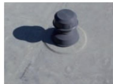
Details are integrated securely and seamlessly into the surface using liquid applied waterproofing. Fittings are not required
