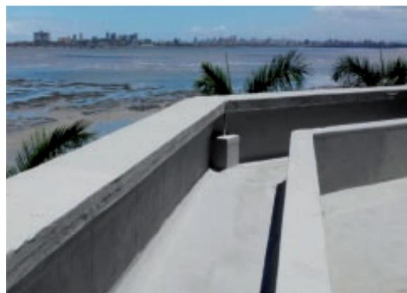
The roof above the server rooms was applied with KEMPEROL®. It protects the concrete structure and provides a barrier against salt water.
